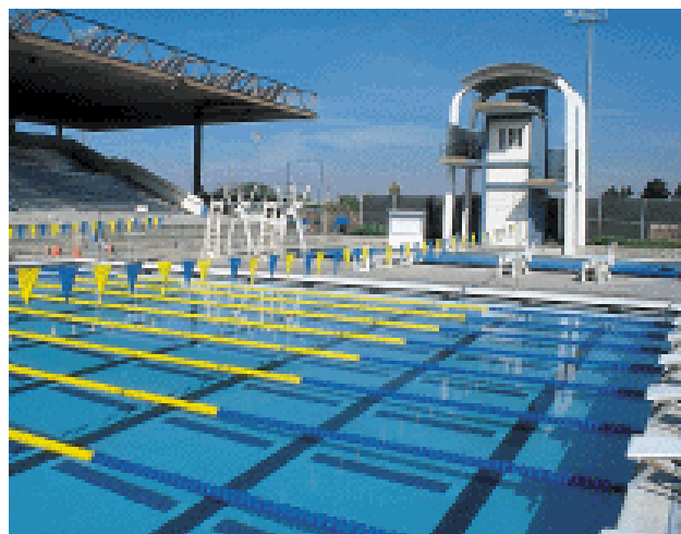
Grandstands and Pool
